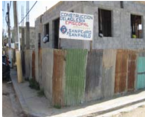
The construction site.
